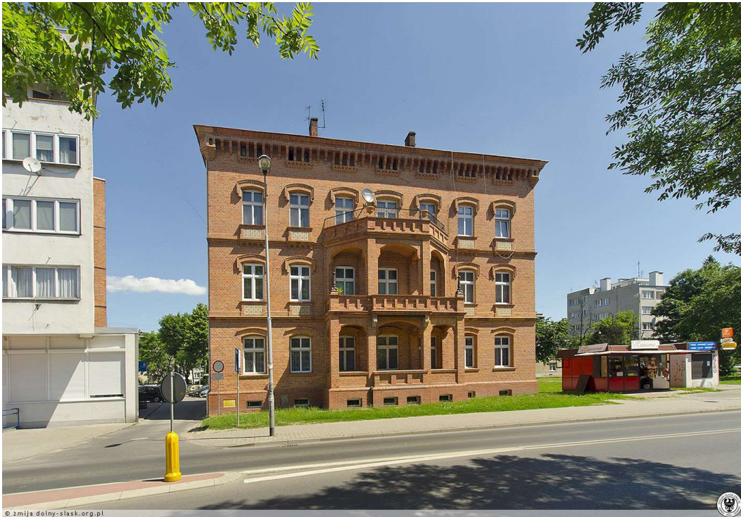
The house at Reja 14–15 in Oleśnica (formerly Bahnhofstrasse in Oels) 175
